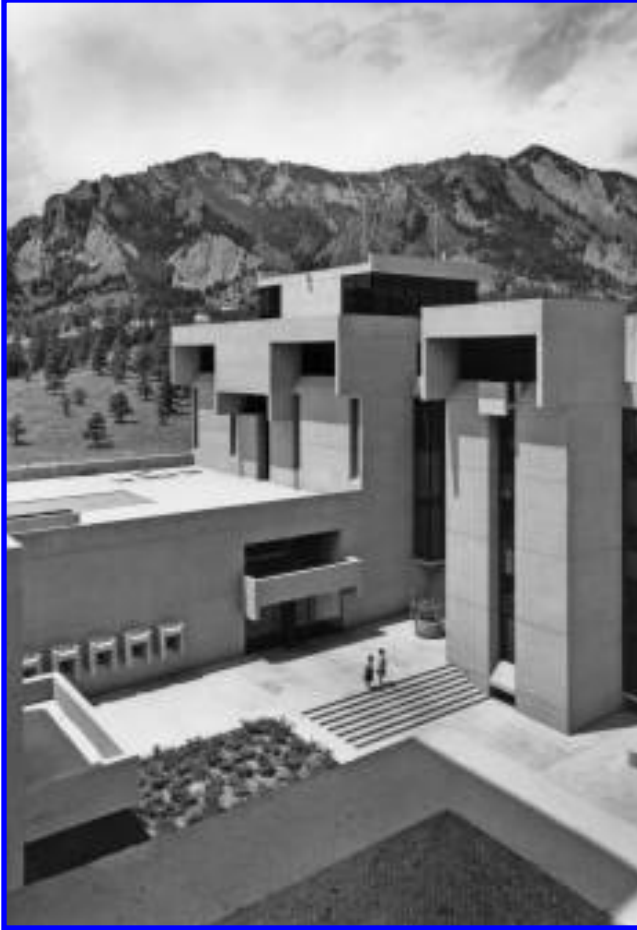
FIG. 2 North Tower of Mesa Lab. Notice the hoods at the top of the towers, above the entrance, and along the row of small windows. The penthouse laboratory and the clutter of antennas that bothered Pei are clearly visible. Notice also the vertical orientation, the actual scale (as measured by the figures at the base), and the “crow’s nest” at the top of the tower. Source: Ezra Stoller, Esto Photographics Inc.
