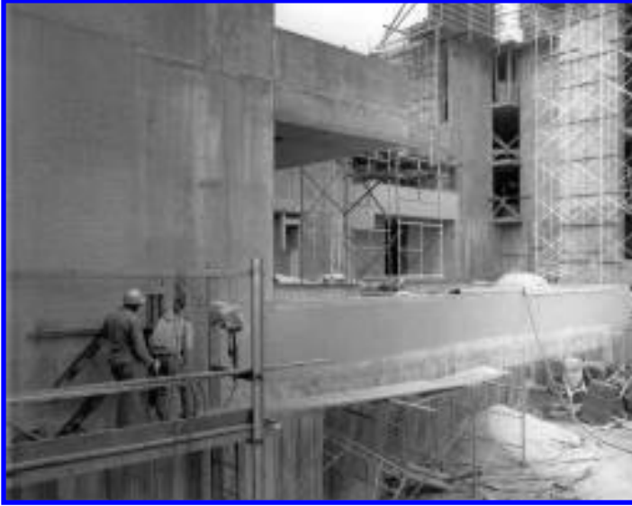
FIG. 3 NCAR's Mesa Laboratory under construction. Workers at the lower left are bush hammering the concrete for a uniform texture. Compare finished concrete with rough form finish to the right. Source: Martin Eby Construction.
